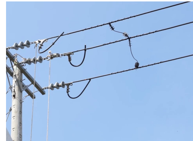
The two components of the cable support safety device are attached to the power lines.
